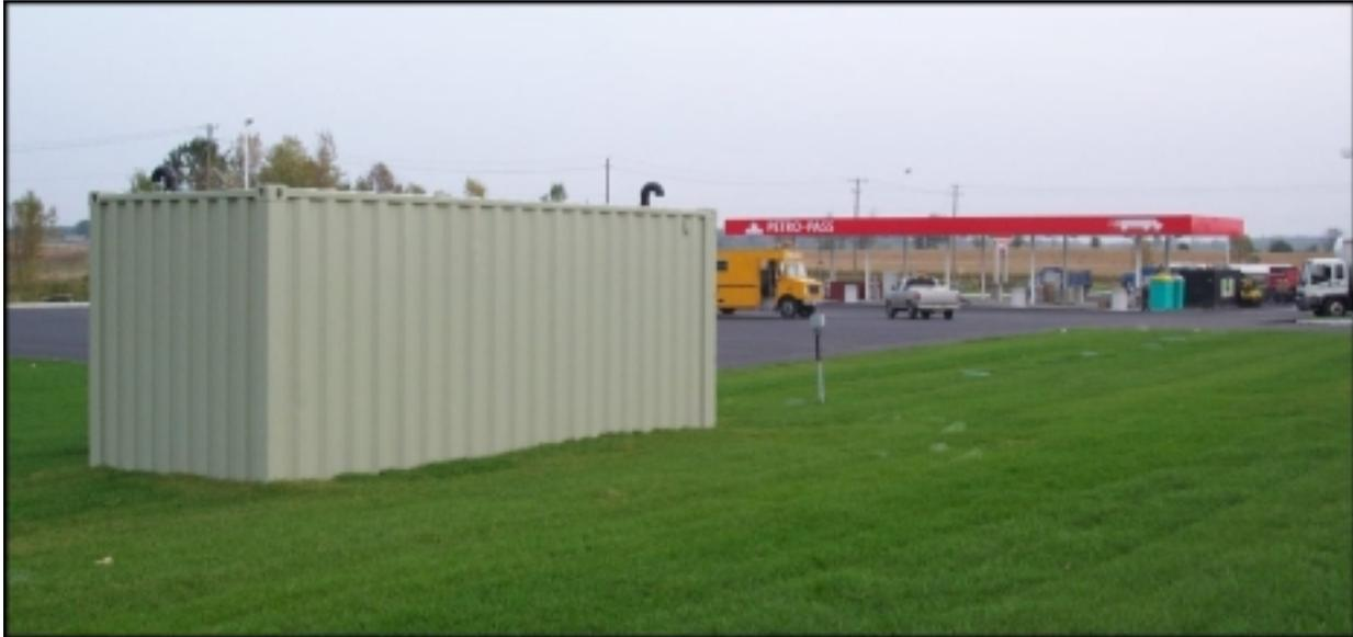
**Figure 2. Waterloo Biofilter SC-20 shipping container at a truck stop, capable of treating 15-20 m<sup>3</sup>/day wastewater. Buried pump and septic tanks are in background.**
