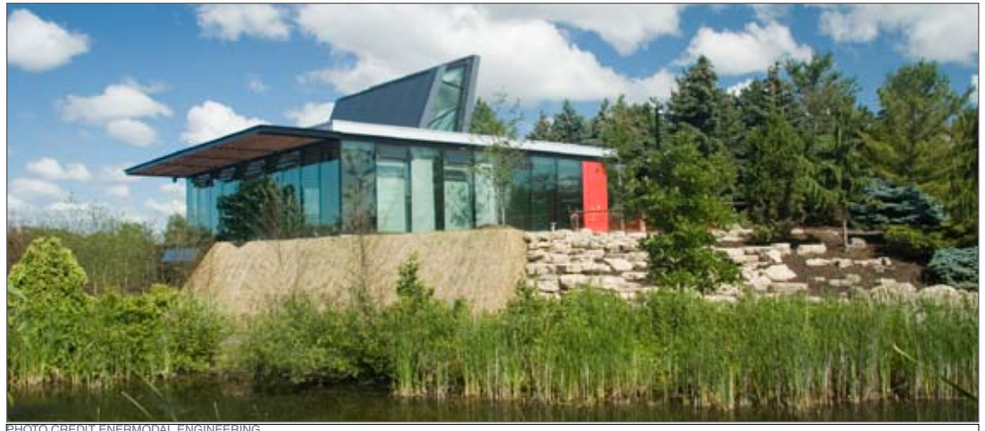
PHOTO CREDIT ENERMODAL ENGINEERING
