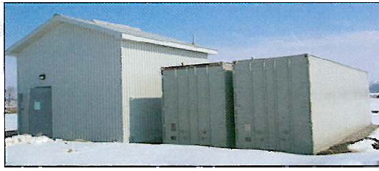
Figure 4. Treatment plant consisting of two SC-40 Biofilter units adjacent to the building housing the MS Filter
