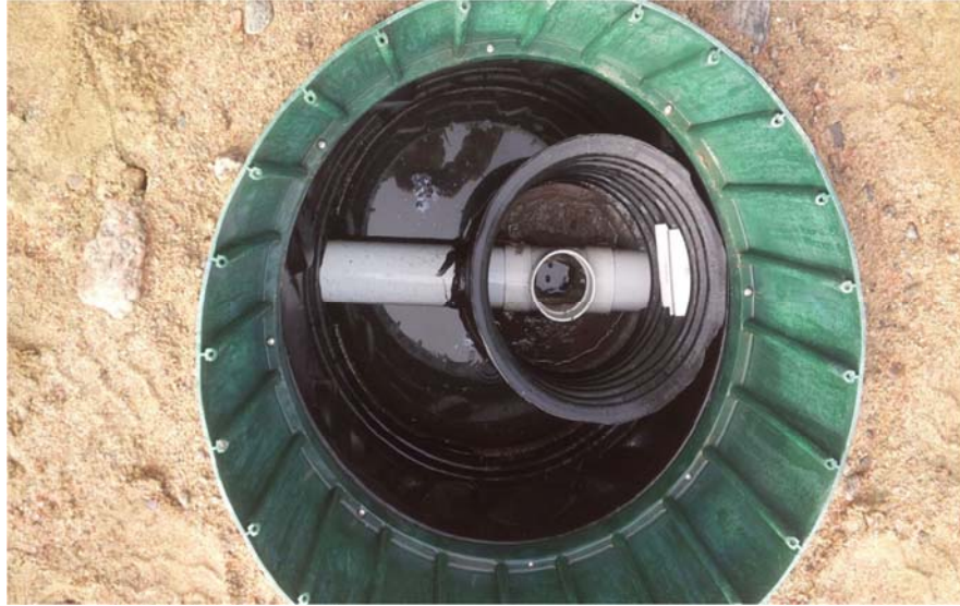
Figure 4b. In comparison, the InnerTube digester has insufficient solids to pump out and effectively no scum layer.
