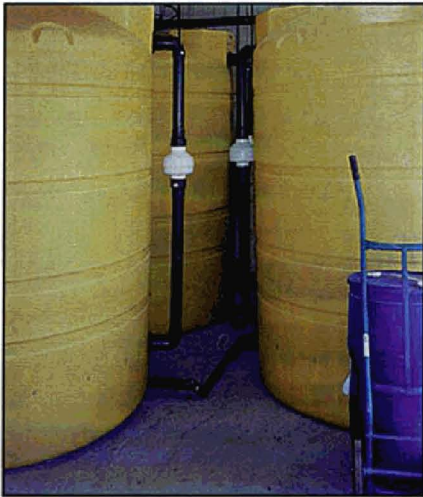
Figure 2. Waterloo Biofilters housed in portable polyethylene tanks 2.4 m diameter by 2.4 m high with controlled air flow using corrosion-resistant fans, each suitable to treat 5000 L/d.
