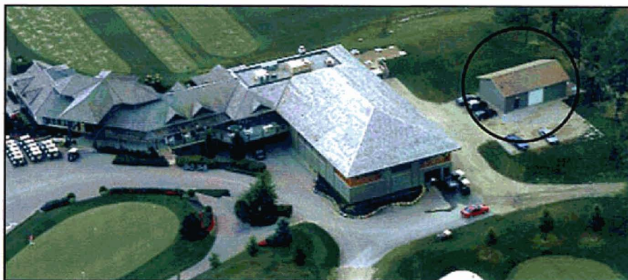
Figure 1. Aerial photograph of Blue Springs golf club showing attractive garage-type building (circled) housing the sewage treatment plant.
